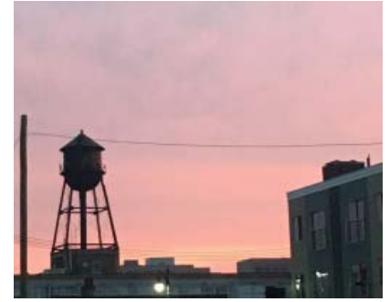
Right: Water tower on top of the Canfield Loft
