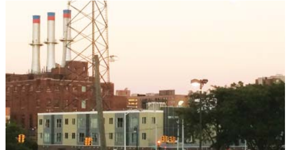
Right: New businesses revitalizing Midtown next to Detroit Thermal LLC on Woodward and Willis
